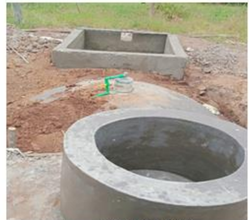
Source: KENPRO, 2021 Field fixed dome biogas digester system
